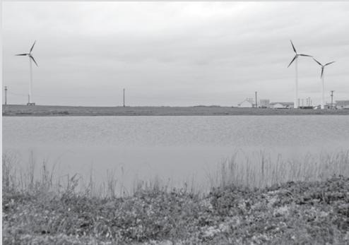
*Kasigluk has three Northwind 100 100-kW turbines with a generating capacity of 300 kW. Total wind-diesel generating capacity is 1,624 kW. Power is also provided to the community of Nunapitchuk through a distribution intertie.*
