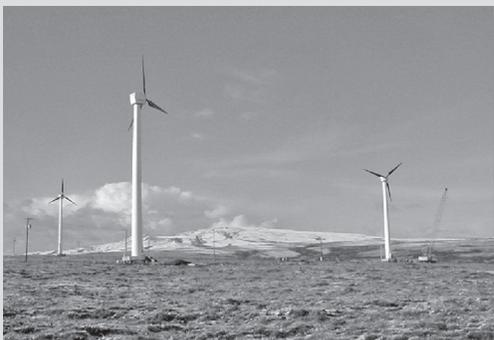
*Toksook Bay has three Northwind 100 100-kW turbines with a generating capacity of 300 kW. Total wind-diesel generating capacity is 1,618 kW. Power is provided to the community of Tununak through a distribution intertie. A tieline is also being built between Toksook Bay and Nightmute.*
