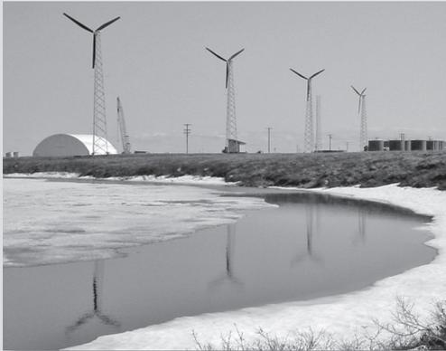
*Selawik, AVEC's first wind farm, has four AOC 65-kW turbines with a generating capacity of 260 kW. Total wind-diesel generating capacity is 1,647 kW.*
