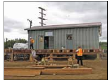
New Stuyahok's power plant was re-located.
