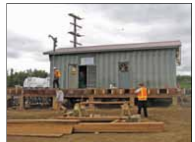
New Stuyahok's power plant was re-located.
