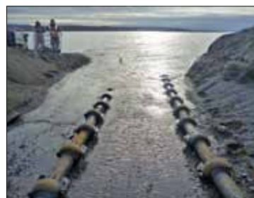
The ends of the Brevig Mission-Teller submarine cables are covered by protective armor.
