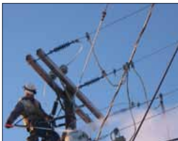
Sam Lindquist powerwashed Savoonga's storm-damaged facilities.
