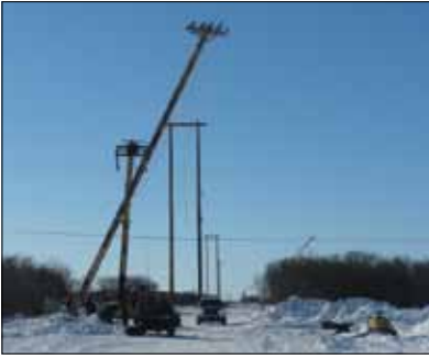
Crews working on the Emmonak - Alakanuk intertie.
