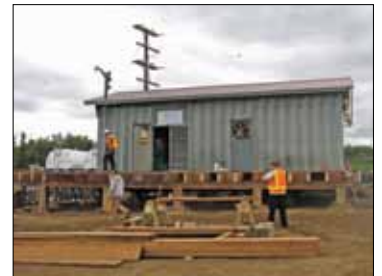
New Stuyahok's power plant was re-located.
