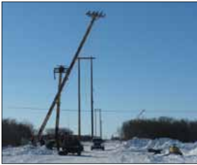
Crews working on the Emmonak - Alakanuk intertie.
