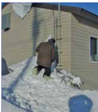
Some meters buried by snow had to be shoveled out.
