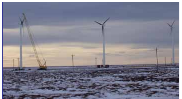
Quinhagak's three new Northwind 100 kW wind turbines.
