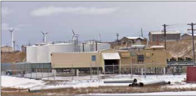
Chevak's new power plant, bulk fuel tank farm and wind turbines.
