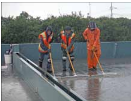
Local residents were hired to help with the construction projects.
