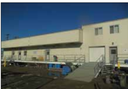
Emmonak's new power plant.
