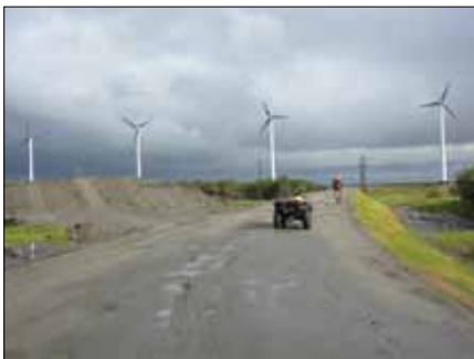
Emmonak's four 100kW wind turbines also provide power to Alakanuk via an intertie.
